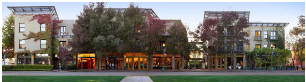
An example of a single mixed use project with varied massing connected by a datum of shade canopies, awnings, trellises, and storefront lintels (top edges). This complex is approximately the width of a 6th street block frontage. This example uniquely represents a national folk architecture with elements of early 20th century modern.
