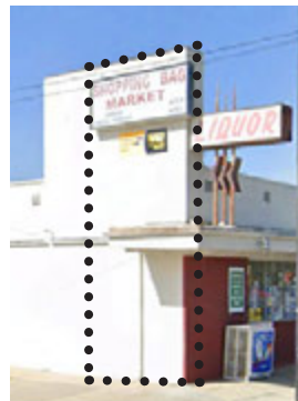
Example of parapet extension on historic building in Beaumont with bounding box for blade sign conformance.
